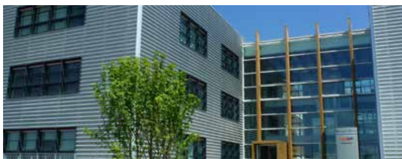
Energy Park Building 4 Vimercate - MI
